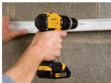
The Wall Dog Screw works very effectively straight into timber and plasterboard where its wide and sharp flutes easily self-drill their way in. They also work well directly into Thermalite blocks and some of the softer brick and even concrete block types. Harder bricks and dense concrete blocks are best drilled out first with a 4mm pilot hole to 35mm depth. The Wall Dog Screw will then pull in tightly to give a good firm fixing.
